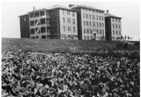
Picture of the old hospital and garden area, from the Glenrose archives.
